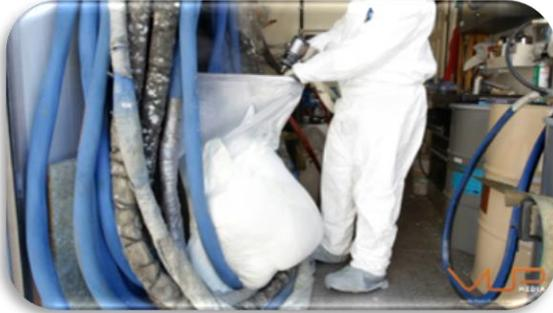
**Always perform a test spray** into a trash bag first to check for mix and rise before installation in walls.
