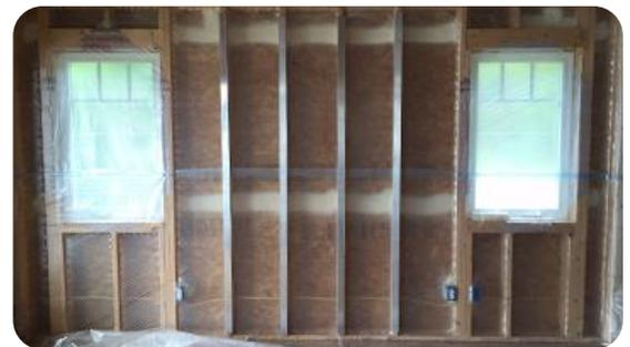
Cap fixture channels are 90" long to fit just inside a standard 8' stud cavity. Use the 72" long cap fixture channels above electrical receptacles on standard 8' stud cavities. Use the 90" cap fixture angles on the ends of walls and on double stud cavities.
