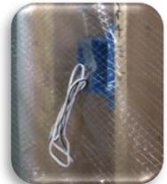
Check to make sure electrical wires have been pulled through membrane before beginning installation of foam.
