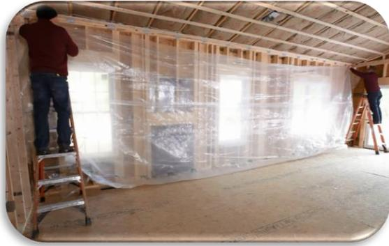
**To begin installation**, stretch the membrane down over the cavity making sure to pull any wires out through it and staple it in place as follows using a Speed Stapler.
