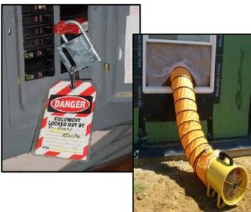
**Use Lock Out / Tag Out** program to ensure HVAC equipment cannot be operated during the spray foam process. For added safety, turn off all power.
