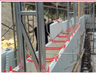
The Quad-Lock Insulated Concrete Forms (ICFs) are extended to prepare for the GacoPolyFoam CF200
