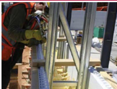
GacoPolyFoam CF200 is poured between two 3" thick Quad-Lock Insulated Concrete Forms (ICFs)
